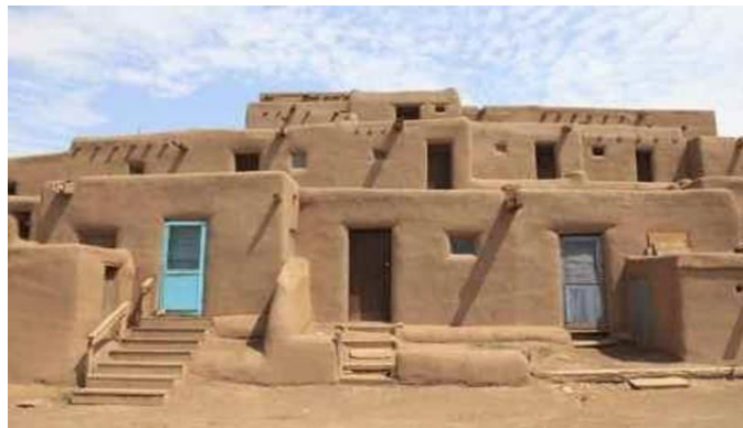
Fig 1: Adobe made Structure
