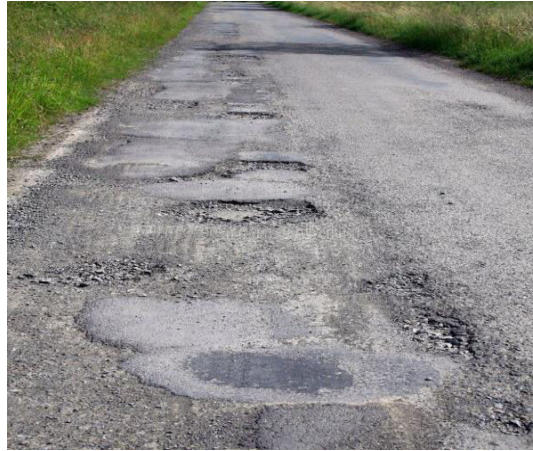
Figure –Patching Of Pavement
