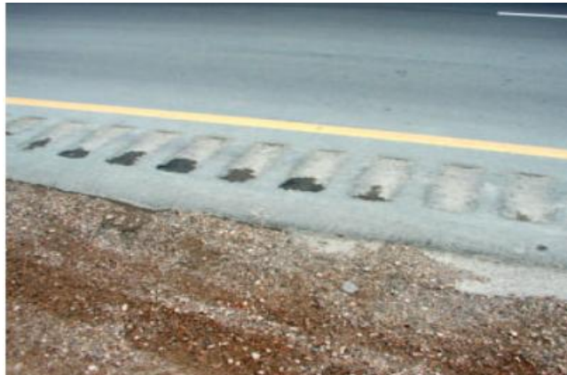
Fig3: Milled Rumble Strip side of the road
