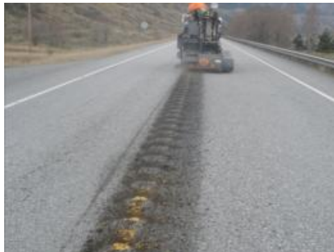
Fig 2: Grinding CLRS
