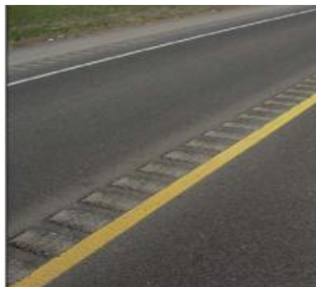
Fig 1: Image of milled centreline rumble strip (CLRS)
