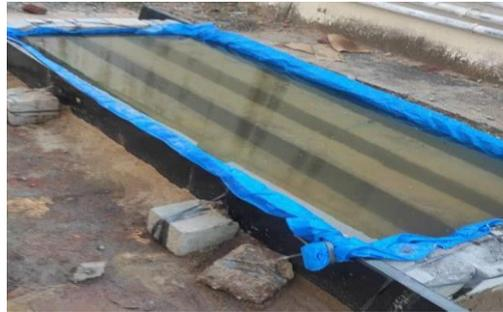
Fig.2 curing of beams into water
