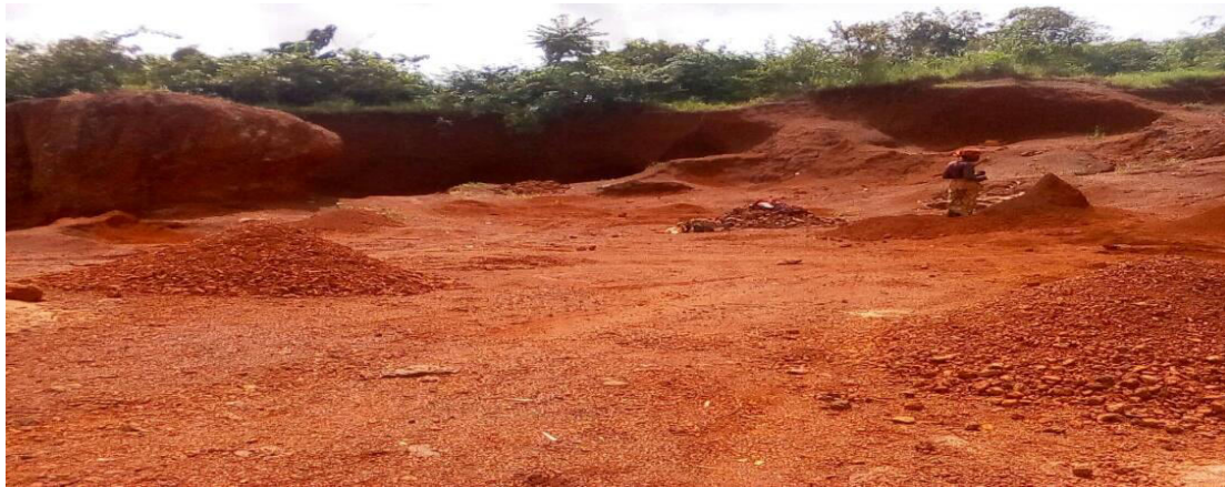
Plate I.: Laterite borrow pit at Ejule, Kogi State Nigeria.
